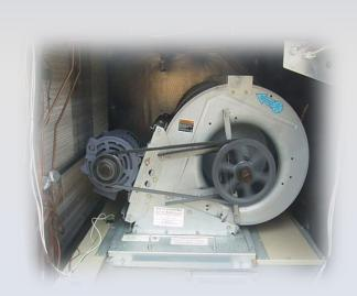
$$PD_2 = PD_1 \times \left(\frac{CFM_2}{CFM_1}\right)$$
