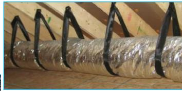
Kinks in the ducts require additional support. When thin materials such as plumbing strap or wire are used for hanging, the duct becomes choked at this point. In severe situations, wire can cut into the duct causing severe air leakage into unconditioned areas of the building.
