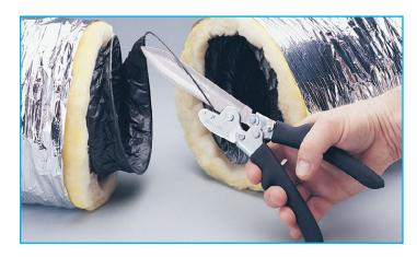
We've removed up to three additional feet of core during many of our duct renovations that would have been missed with a visual inspection. As a result we've measured airflow increases of 30 to 40 cfm on a 6-inch duct by removing excess core.
